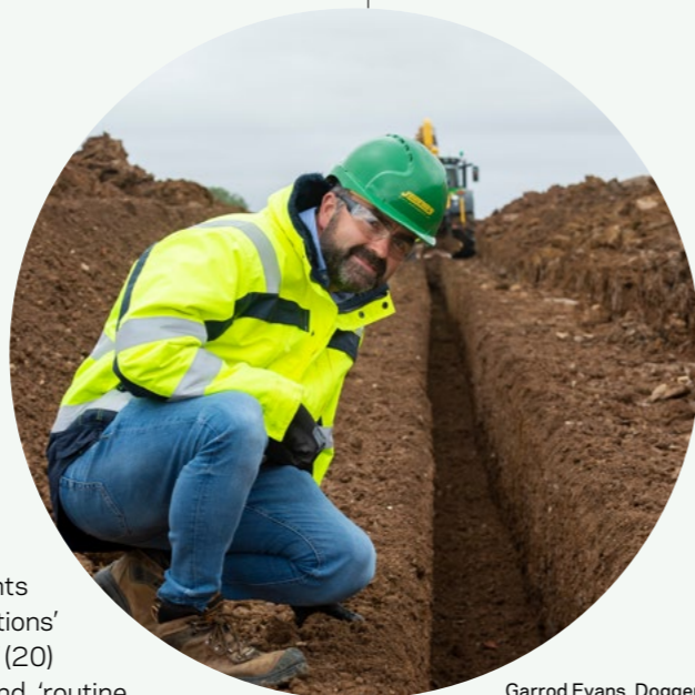
Garrod Evans, Dogger Bank onshore cable works
