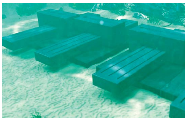
H-WEP 1 layout on the seabed
