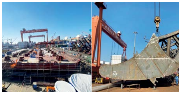
Construction of Wave Energy Platforms
