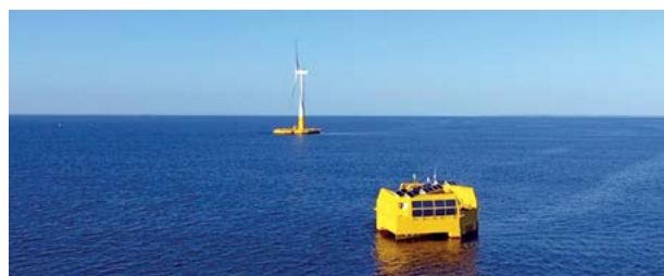
Wavegem hybrid wave-solar platform and Floatgen floating offshore wind turbine currently being tested at SEM-REV (ECN credit)
