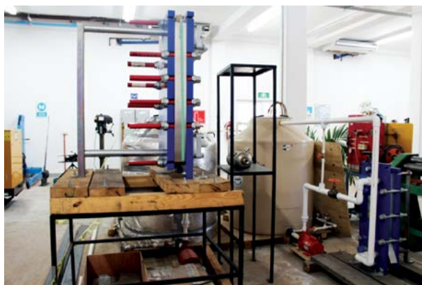
OTEC facility at CEMIE-Oceano
