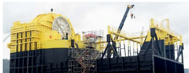
OE Buoy near complete construction at the Vigor yard in Portland, USA
