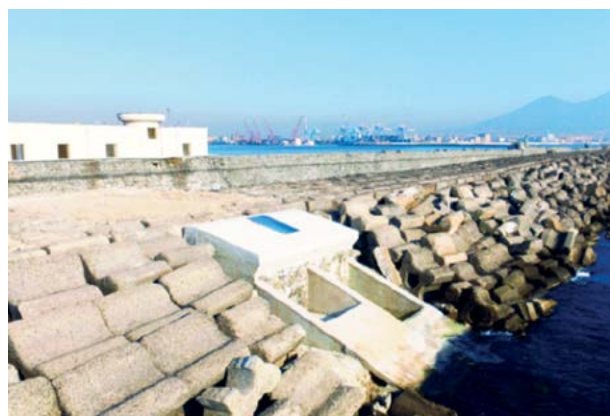
Breakwater equipped with the OBREC prototype in the port of Naples
