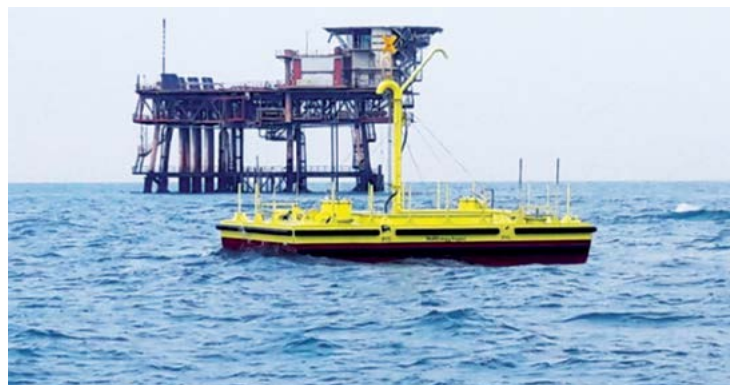
ISWEC installation offshore Ravenna coast
