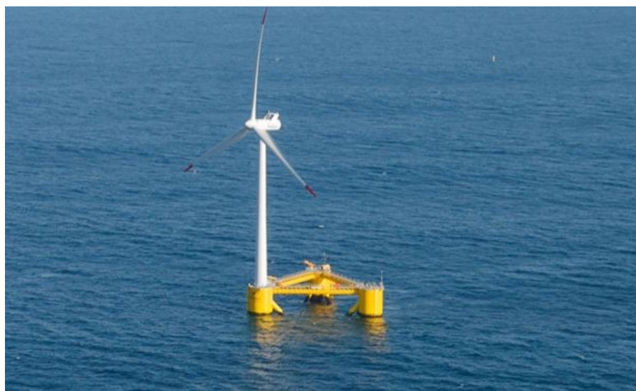
Figure B3. WindFloat I Prototype on station in Portugal—deployed 2011–2016
