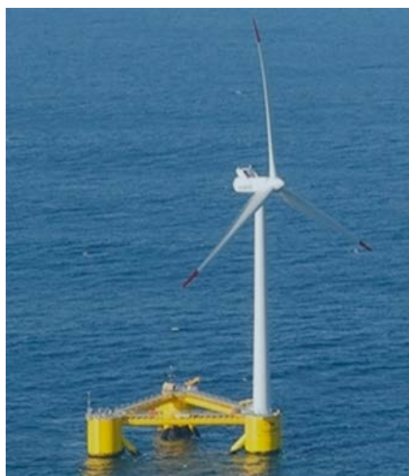
Figure B8. The WindFloat prototype with the substructure technology that will be used to support 6-MW Haliade turbines for the Les eoliennes flottantes du Golf du Lion (Leucate) floating project
