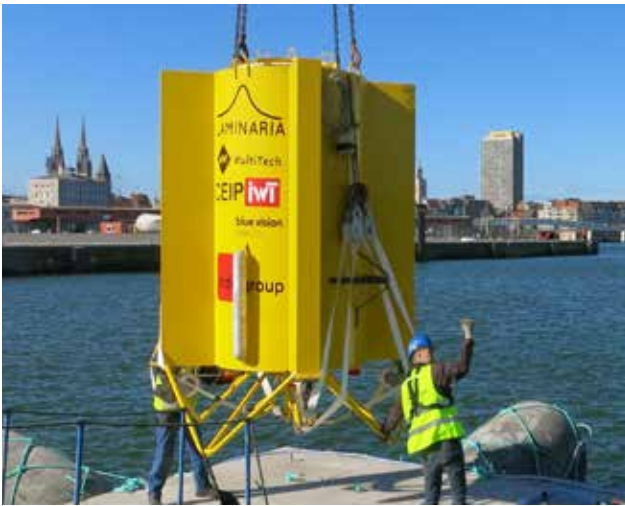
Figure 5. A point absorber WEC (Laminaria).
